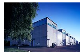
Stadler Stahlguss 120 employees
